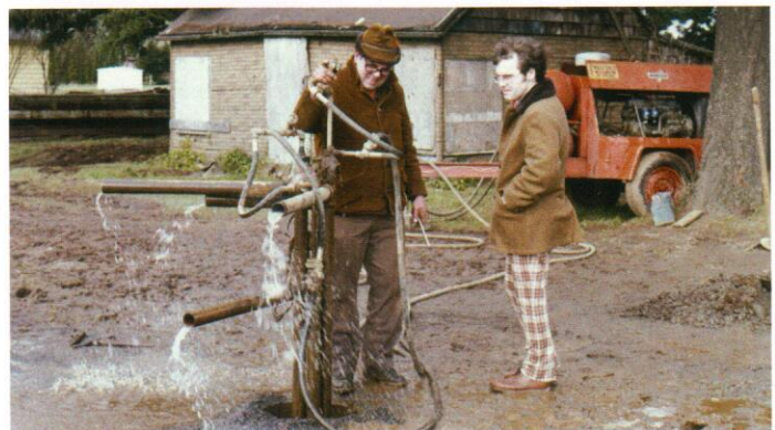
Exploratory well testing in 1976.
