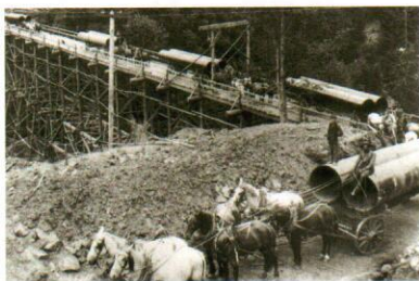
Six-up horse teams and drivers delivering conduit pipe in 1893.
