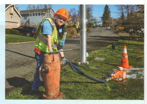
the water mains. This material can impact water quality and cause customers to see discolored water at the tap when it is stirred up by construction or other activities. The high-speed flushing, called unidirectional flushing, scours the insides of the pipes and removes the accumulated materials from the water mains. This routine cleaning improves the health of Portland's system now and ensures the health and integrity of the system for the future.
